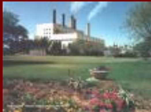
Eshkol power station Haifa
